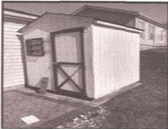
Haven Tree Ct BEFORE.....
